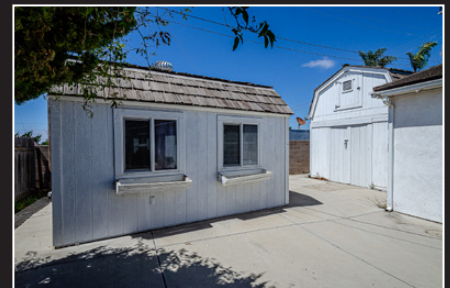
Two Large Sheds in Rear
